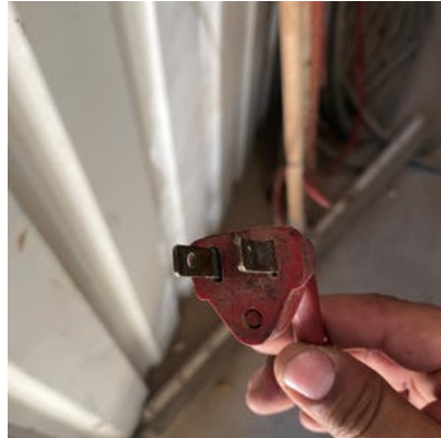
Extension cord missing ground prong.
