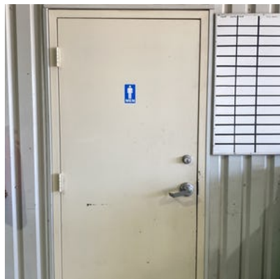
Non-exit properly marked.
