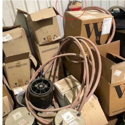
Obstructed path to extinguisher. I discussed the location of this with Rocky and it was removed. The other three extinguishers in the shop satisfy the 75 ft travel distance required.
