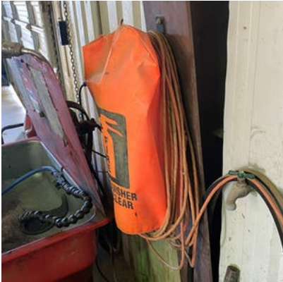
Same extinguisher had extension cord wrapped around.
