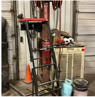
Obstructed path to extinguisher / Improper storage location for propane tank
