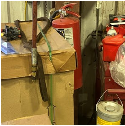
Material storage in front of extinguisher.
