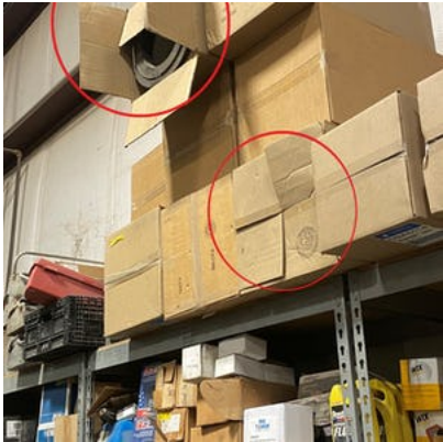
Opened-end boxes facing personnel travel area. Need to be placed upright or facing inward towards wall.
