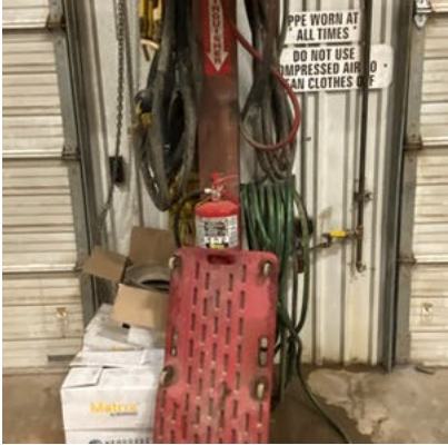
Obstructed path to extinguisher / Slip hazard with excess water from faucet
