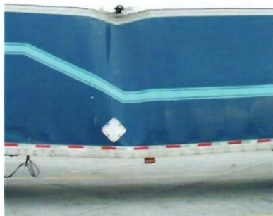
a. (1) Broken Upper Rail
