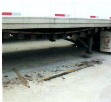
c. (1) and (2) Protruding Freight and Sagging Crossmembers
