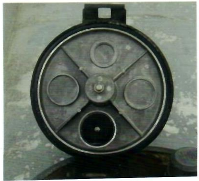
d. Open Manhole Cover
