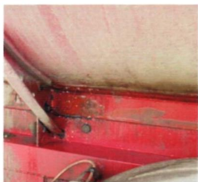
e. Leaking Cargo Tank
