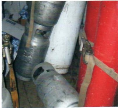
a. HM/DG Not Properly Secured
