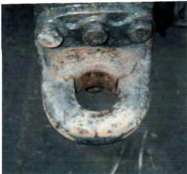
d. (3) Welded Repair to Drawbar Eye
