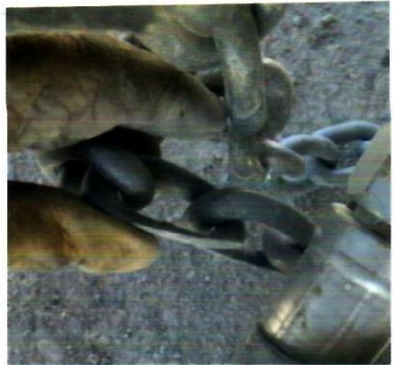
f. (4) Excessive Wear
