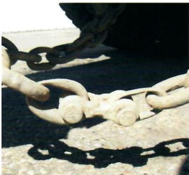
f. (4) Excessive Wear
